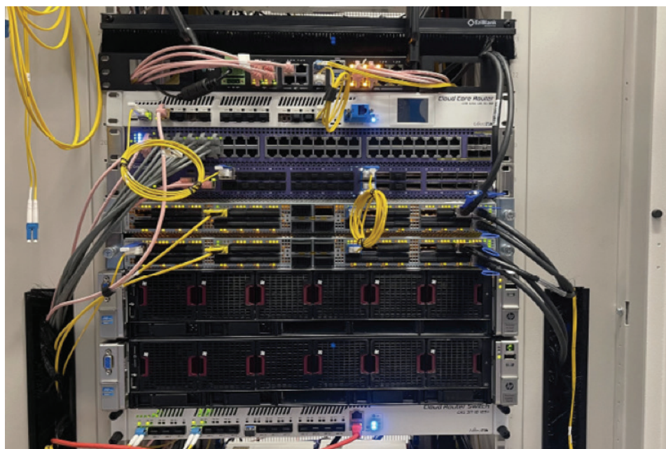
Image: The Nodegrid Gate SR sits at the top of the rack to provide in-band and out-of-band networking Source: IAA supplied
